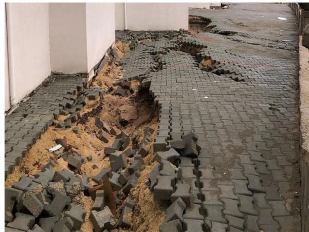
**Figure 3.** Soil response indicating bearing capacity loss.
