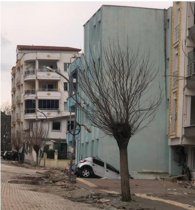
**Figure 2.** Heavily settled building due to liquefaction.
