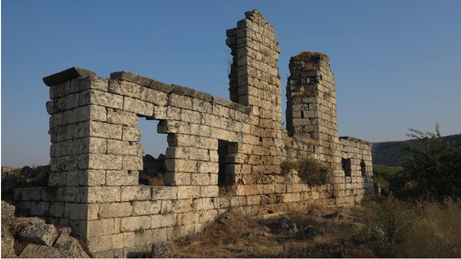
F. 16: The eastern facade of the North Church, view from the southeast (A. Tiryaki, 2022)
