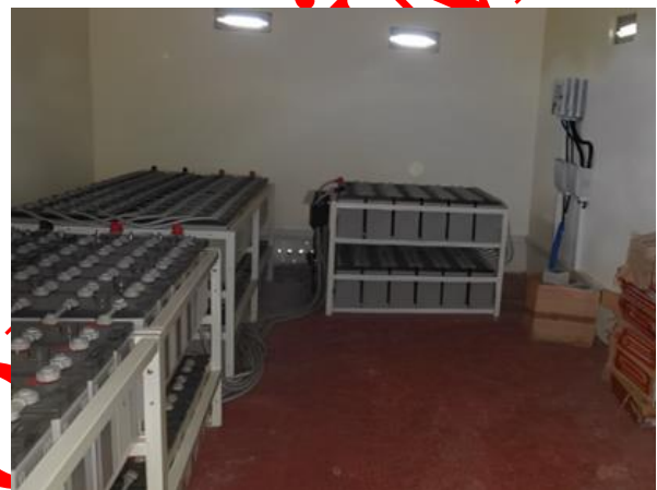
Figure 4. The powerhouse installed in Gagrawara
