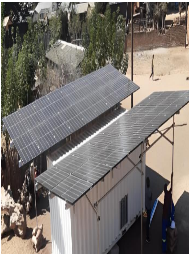
Figure 6. In Gagrawara, solar panels have been set up to form a mini- power plant that generates and distributes electricity
