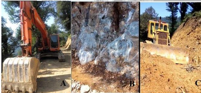
Figure 2. Road profile and construction machines A) Doosan excavator, B) hard rock trench, C) Komatsu bulldozer in soft (soil section) layer
