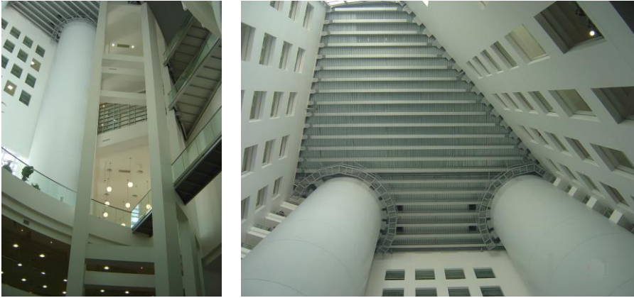
Figure 5. Several views from atrium (from the author's archive).
