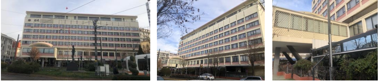
Figure 15. Eskişehir Porsuk Hotel [20]
