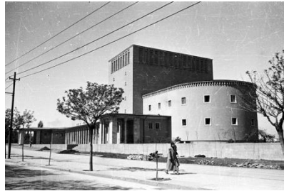
Figure 3. Opera House after conversion [19]
