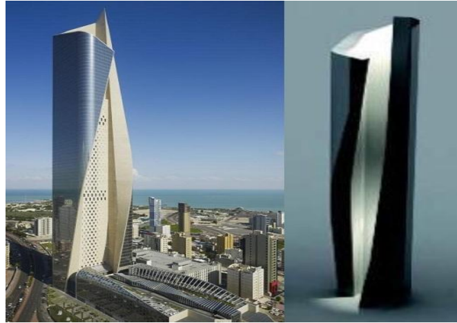
Figure 21. Al Hamra Tower (URL-34; URL-35).
