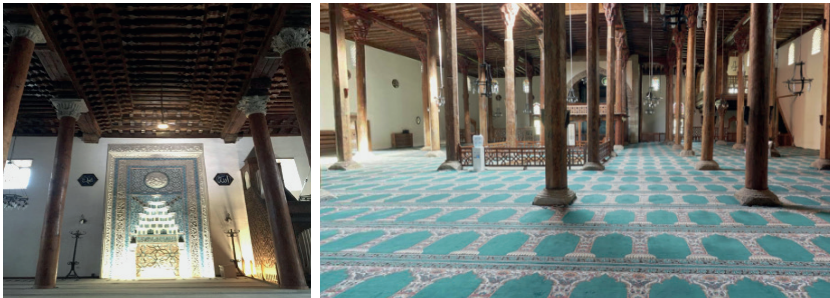
Figure 4 Timber ceiling, coloumns and the minber in Aslanhane Mosque (Onur Şimşek)
