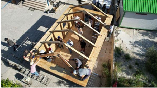
Figure 10. Dismantling of the prototype to be transported to Hatay after the opening (Günhan, 2023)
