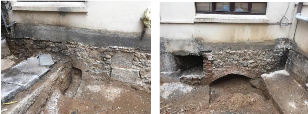
Figure 18. In the inner courtyard, two arches and galleries (2023 Restoration)
