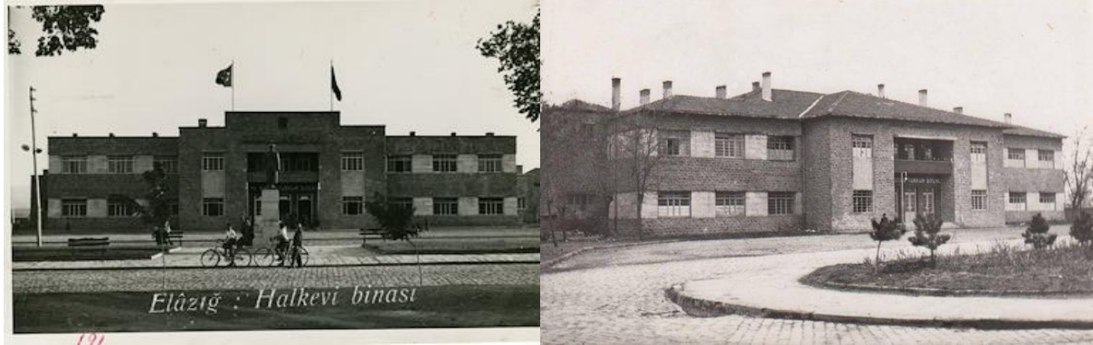
Figure 18. The entrance facade of the Elazığ People's House [20]
