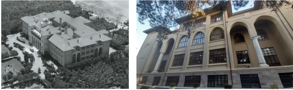
Figure 16. a) Gazi Education Institute [68], b) Gazi Education Institute Side Facade (by author)
