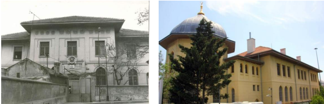
Figure 5. a) Reşadiye School Facade Photo [23], b) Reşadiye School Facade Photo [55]
