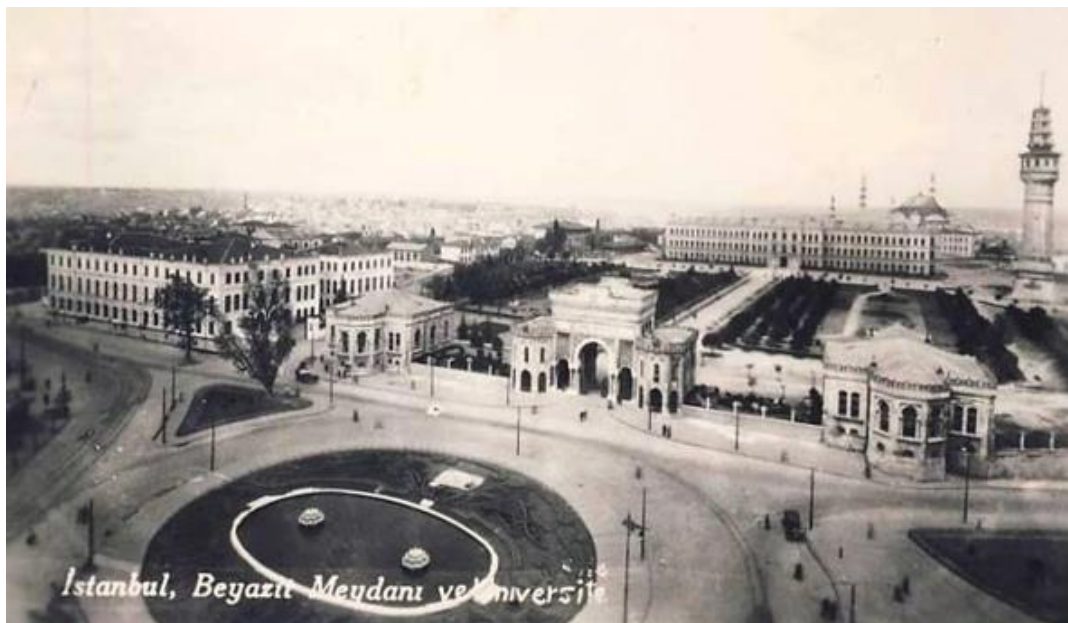
Figure 10. The fountain pool condition of the square, 1930s (INT-3)
