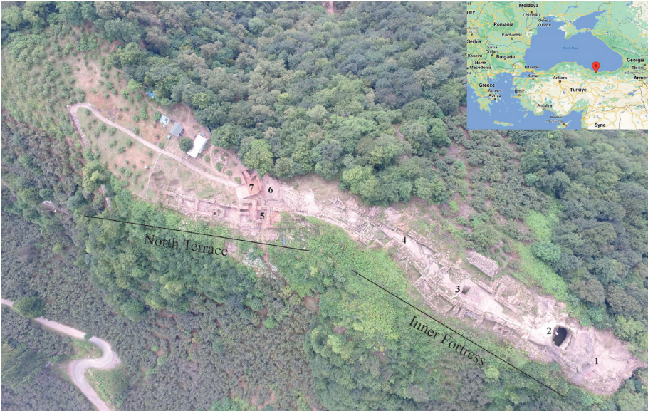
Fig. 1 Aerial photograph of Kurul Kalesi. (© Kurul Kalesi archive). 1. The rock altar and the open-air cult area; 2. The rock reservoir (so-called cistern); 3. The stepped tunnel; 4. Corridor; 5. Niche of Kybele and Kybele cult area; 6. An area covered with stacked stones after losing its cultic function; 7. Dionysus sanctuary.
