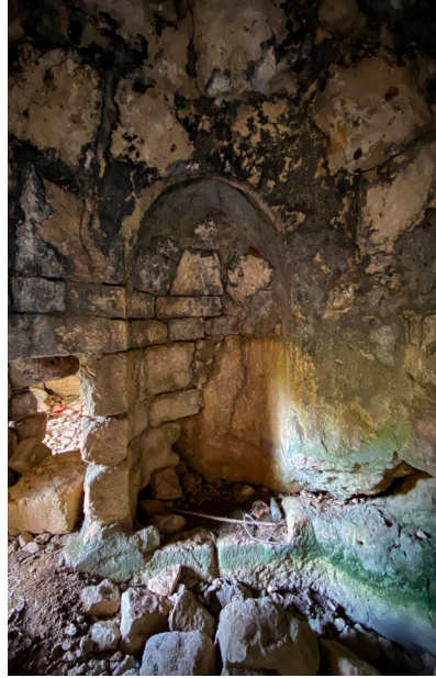
Fig. 13 Apse Details from Space Number 1 in Hasanaliler Church
