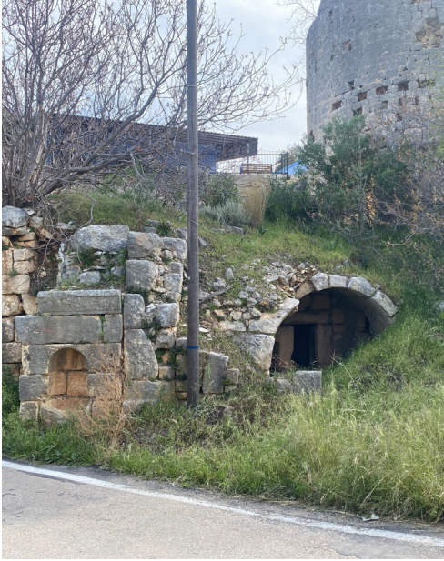
Fig. 12 Bottom Elevation Spaces in Hasanaliler Church
