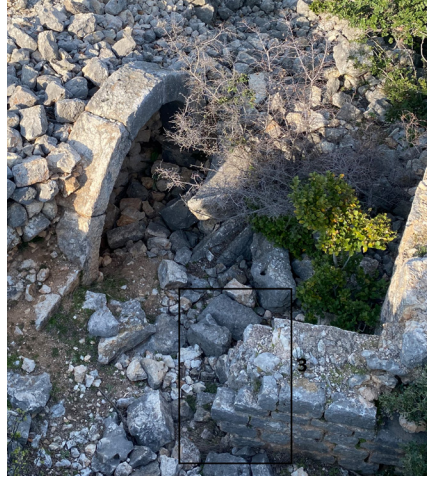
Fig. 11 Wall Detail from Yanıkhan South Church
