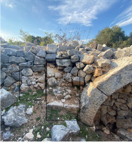
Fig. 10 Wall Detail from Yanıkhan South Church
