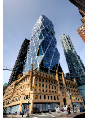
Şekil 14. Hearts Tower, Norman Foster and Partners, New York, 2001, (Doğal Havalandırma, Aydınlatma, Akıllı Kabuk) (Natural Ventilation, Lighting, Smart Shell) (22)
