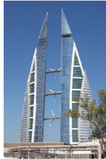
Şekil 23. Bahreyn Dünya Ticaret Merkezi, Atkins 2008, Bahreyn, (Rüzgâr Türbini, Doğal Aydınlatma, Çevre Dostu Malzeme), Bahreyn World Trade Centre, Atkins, 2008, Bahreyn) (Wind Turbine, Natural Lighting, Environmentally Friendly Materials) (36)
