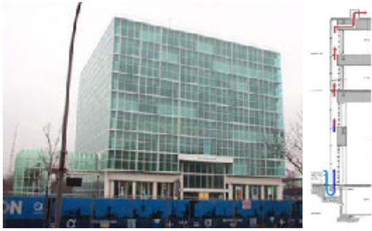
Şekil 18. Occidental Chemical Centre, Canon Design Inc., Mark R. Mendell, 1980, New York, (Çift Kabuklu Cephe Uygulaması) (Application of Double Shelled Wall) (20)
