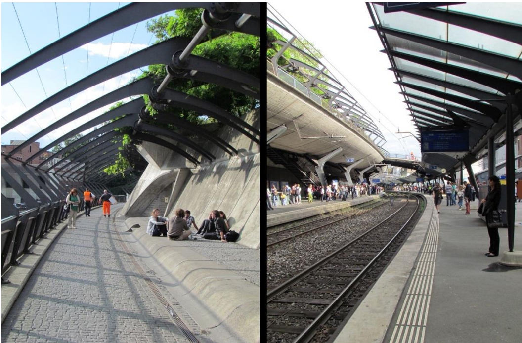
Figure 8. Stadelhofen Station, Different Levels and Materials (Photo taken by the author, 2013).
