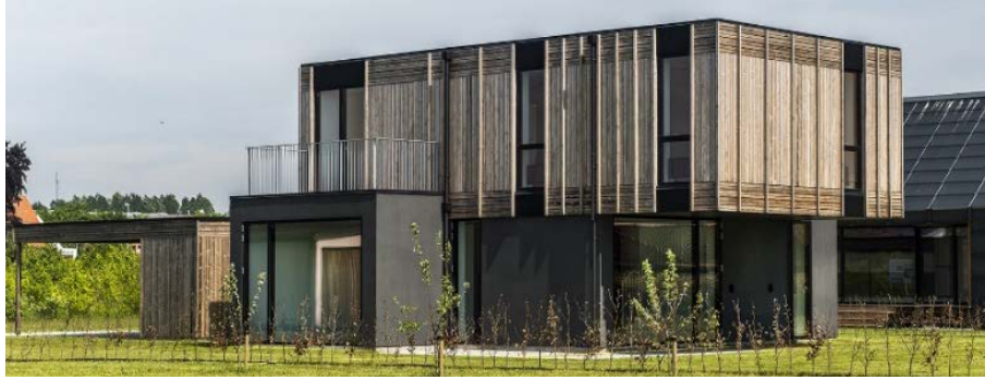
Şekil 6. Henning Larsen Architects, Nyborg Adaptable House (URL- 6)
