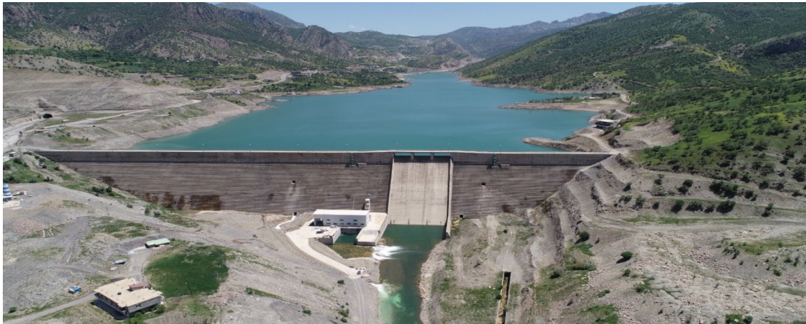
Figure 2. Uludere Dam-Elbi HEPP
