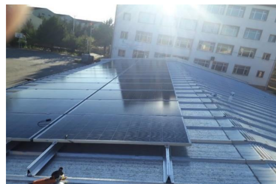
Figure 4. Installation of PV Panels on the roof in 2 chains
