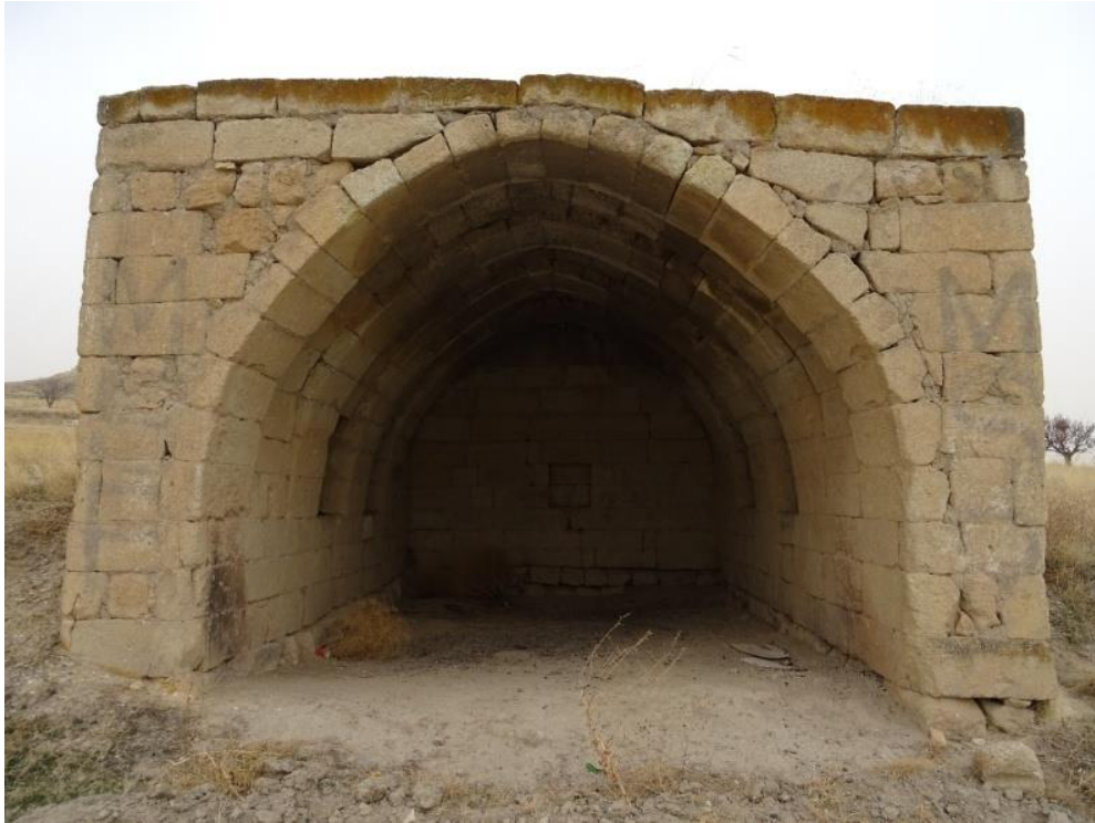
Photo9. Building no. 3621 -Front facade and entrance arch and interior (Tokat, 2021).
