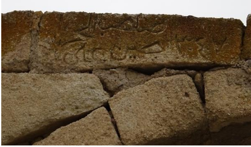
Photo9. Building no. 3621 - Inscription stone on the entrance arch (Tokat, 2021).
