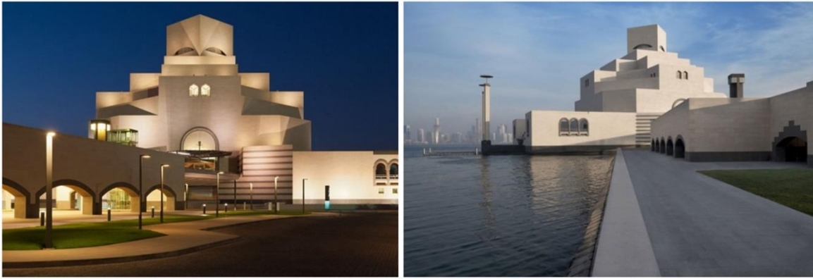
Figure 6. Gradual elevation of the form [49, 59]
