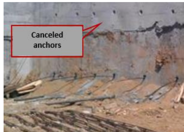
Figure 3. The canceled first row of anchors [5]
