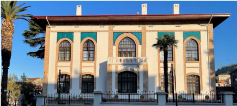
Fig. 7: West Facade General View
