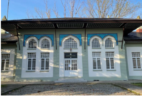
Fig. 17: Edirne-Karaağaç Old Station Building
