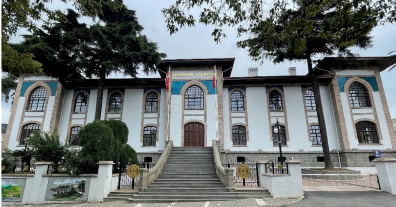
Fig. 5: General View from the Front (North)
