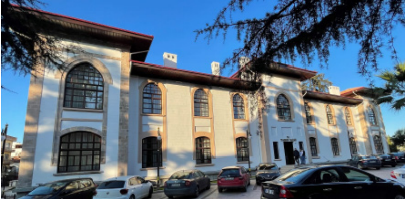
Fig. 6: South Facade General View
