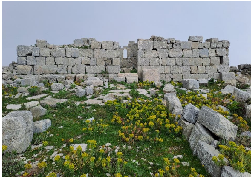
Figure 5: West exterior facade (M. Kaya, 2024)
