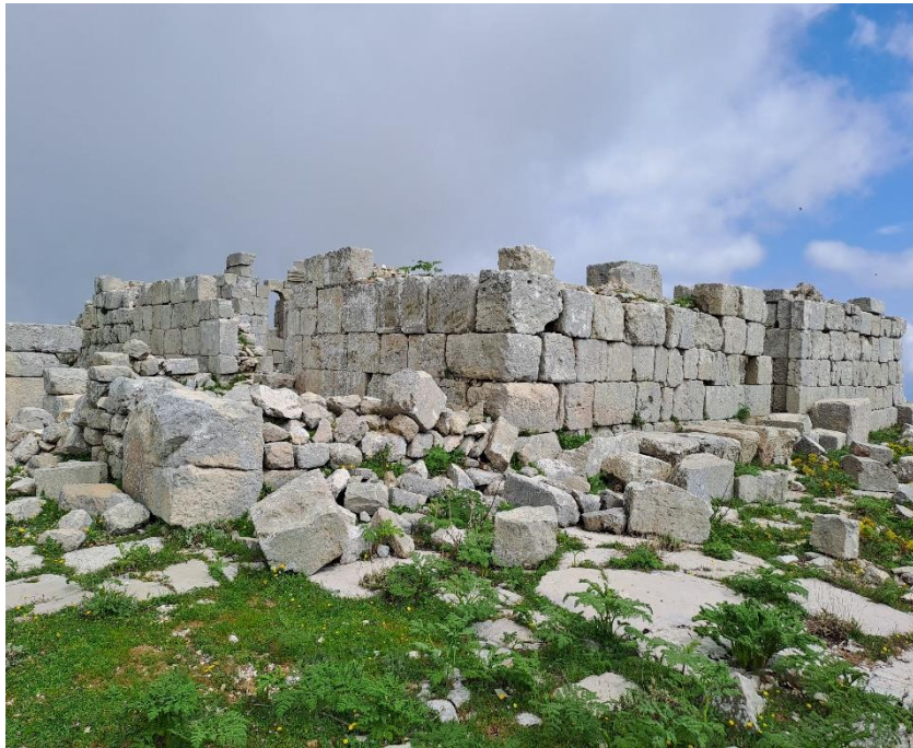
Figure 7: North-west exterior facade (M. Kaya, 2024)
