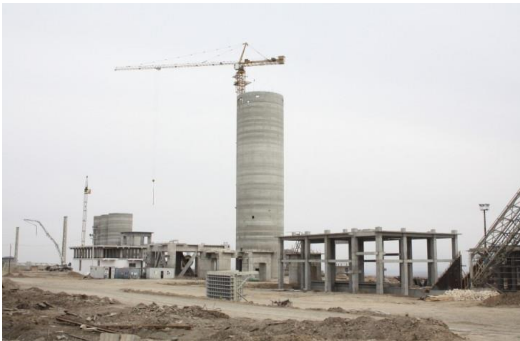
b) A view during construction from east side of the plant
