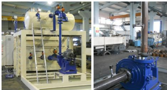
Figure 5. The experimental set-up (left) and the original centrifugal slurry pump(right)
