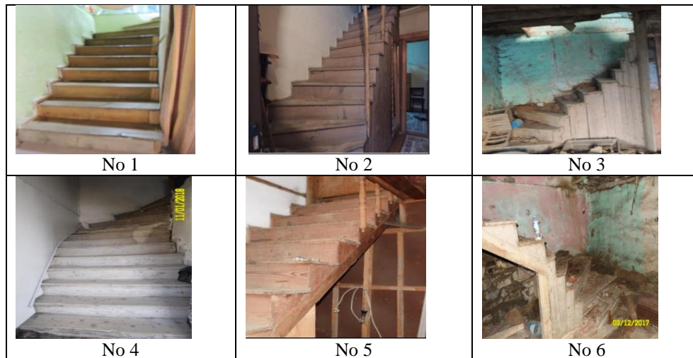
Figure 12. Staircase Images of Houses No. 1, 2, 3, 4, 5, and 6
