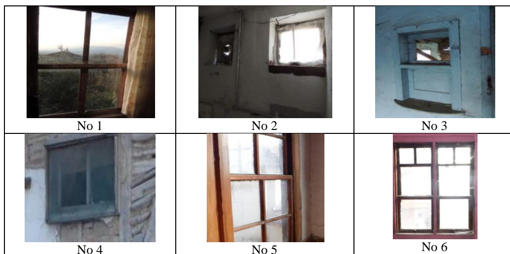
Figure 14. Windows of Houses No. 1, 2, 3, 4, 5, and 6
