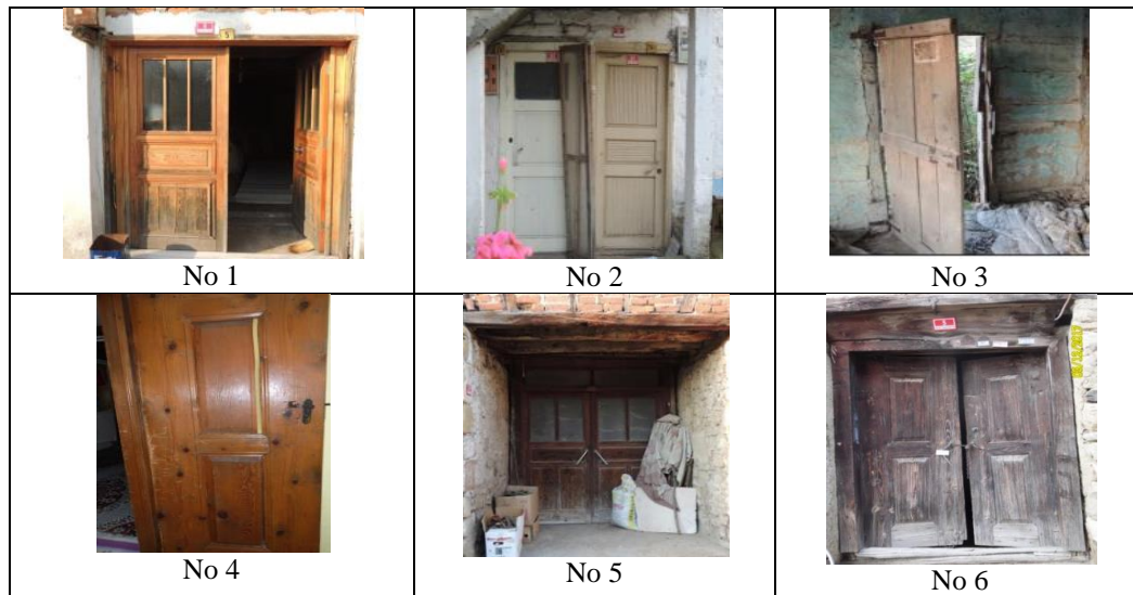
Figure 13. Main Entrance Doors of Houses No. 1, 2, 3, 4, 5, and 6
