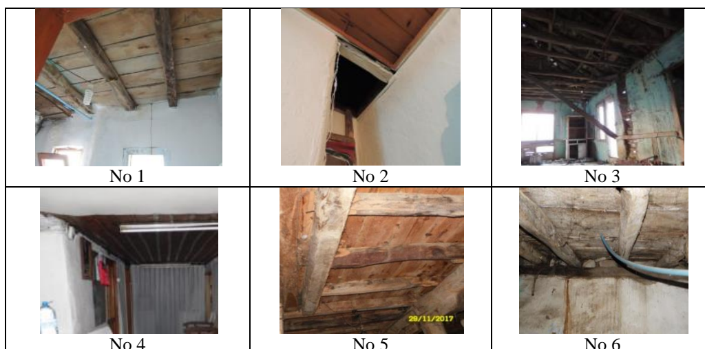
Figure 11. Ceiling Images of Houses No. 1, 2, 3, 4, 5, and 6
