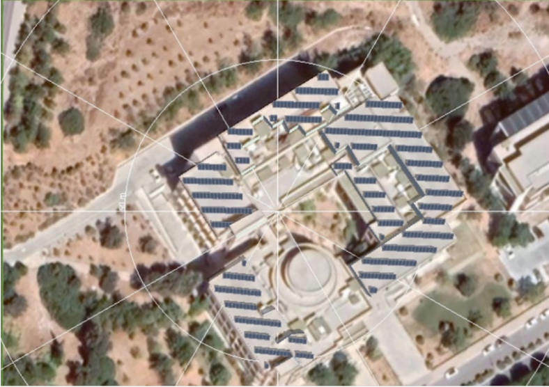
Figure 5. Flat Roof PV Panel Installation by PV-Sol Software
