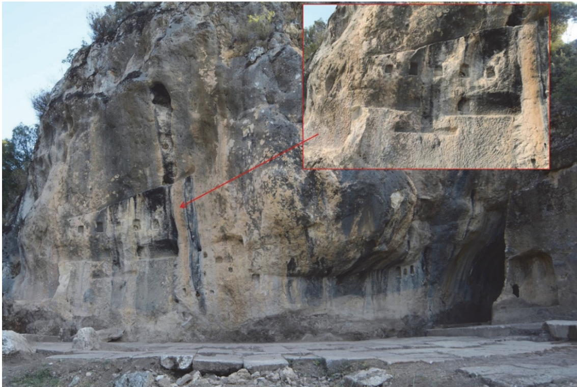
Fig. 27) Beam sockets created to support the roof on the main rock facade surrounding the sacred area from the west and north
