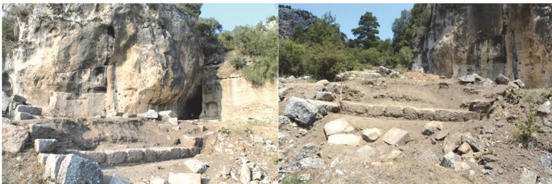
Fig. 9) Sanctuary east retaining wall
