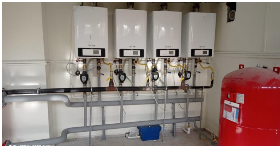
Figure 6. Installation of cascade heating system
