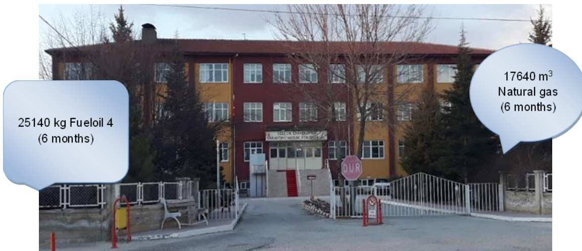
Figure 4. Sarayönü Vocational School and Approximate Resource Usage Amounts
