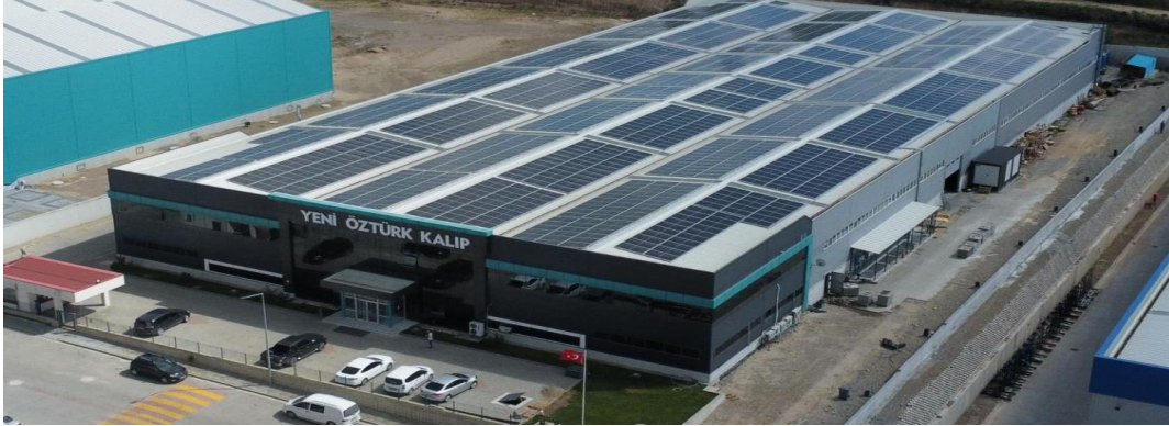
Figure 1: General view of the industrial facility
