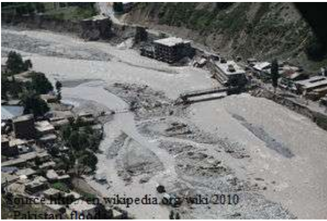
Fig.11 Bridge collapsed during flood 2010 [22]
