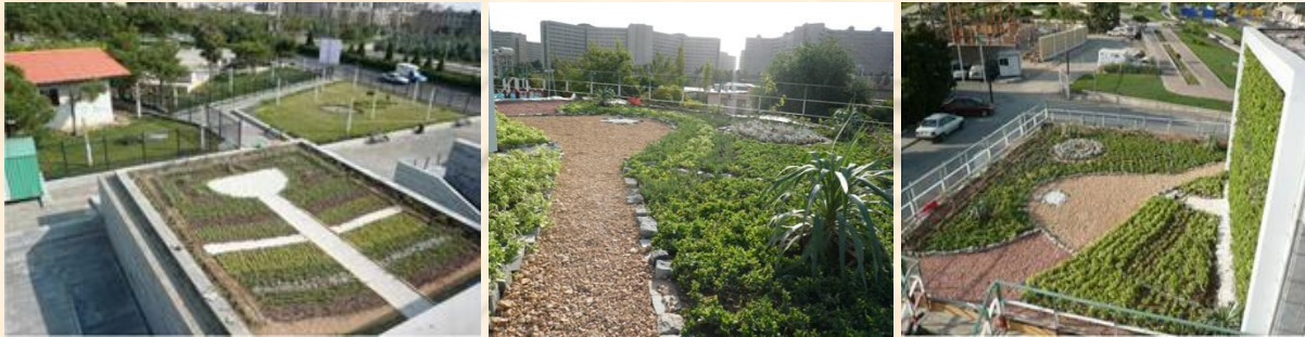
Figure 6. An extensive green roof, Ekbatan green roof project, Tehran (23).
