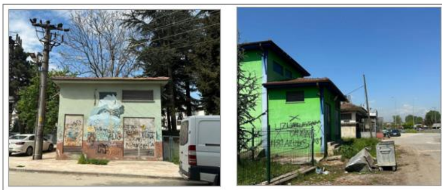
Figure 25. Appearances of transformer buildings located in the working area of Düzce/Uzun Mustafa neighborhood
