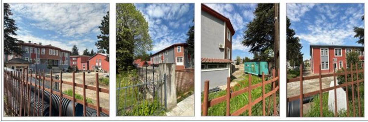
Figure 10. Views of Düzce Vocational High School and its surroundings located in the working area Düzce/Uzun Mustafa neighborhood
