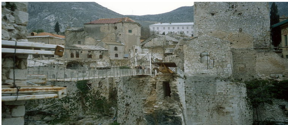
Figure 3. Temporary Bridge After Destruction
