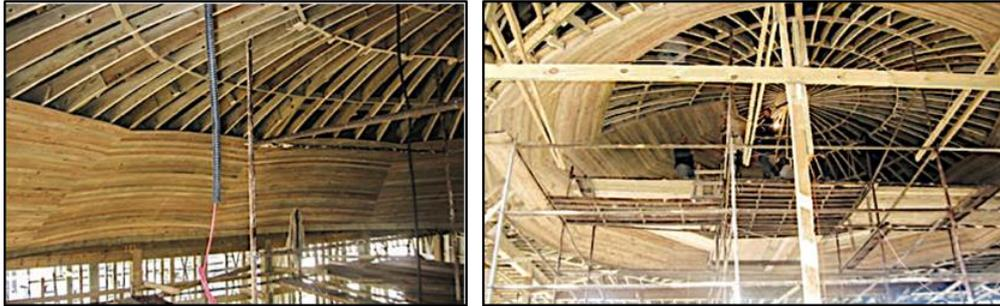
Figure 12. The wooden dome restoration of Yenikapı Semâhane [21]
