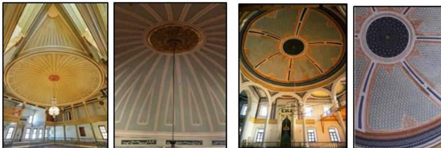
Figure 14. The division of the wooden dome into geometric slices starting from the centre towards the rim in Yenikapı and Gelibolu Semâhanes [7]
