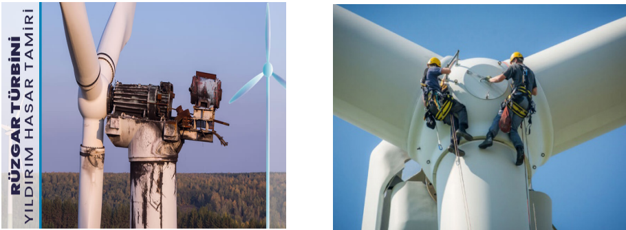
Figure 2. Wind Turbine Lightning Damage & Maintenance (URL-5)
