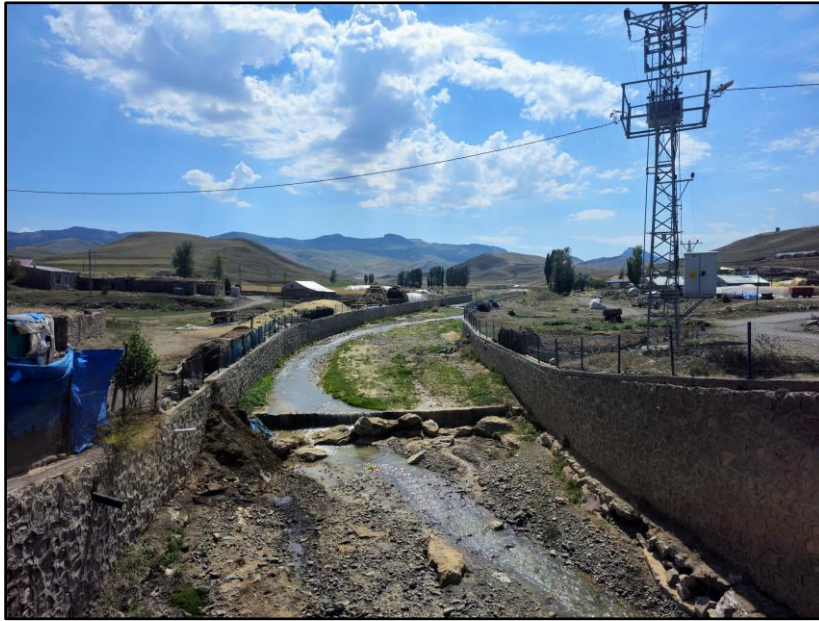
Figure 11: River retaining walls and streambed rehabilitation in Alagöz village.
