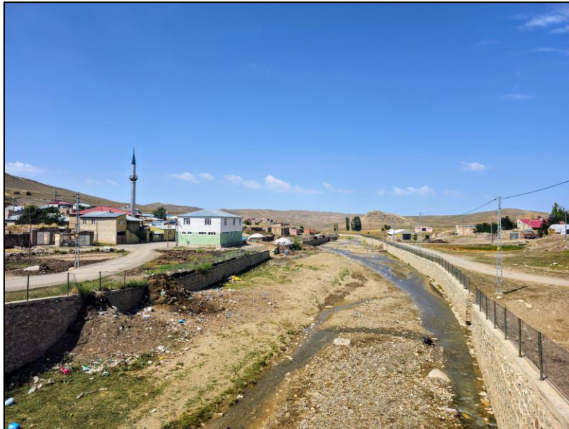
Figure 12: The uncontrolled filling of the riverbed with waste materials.
