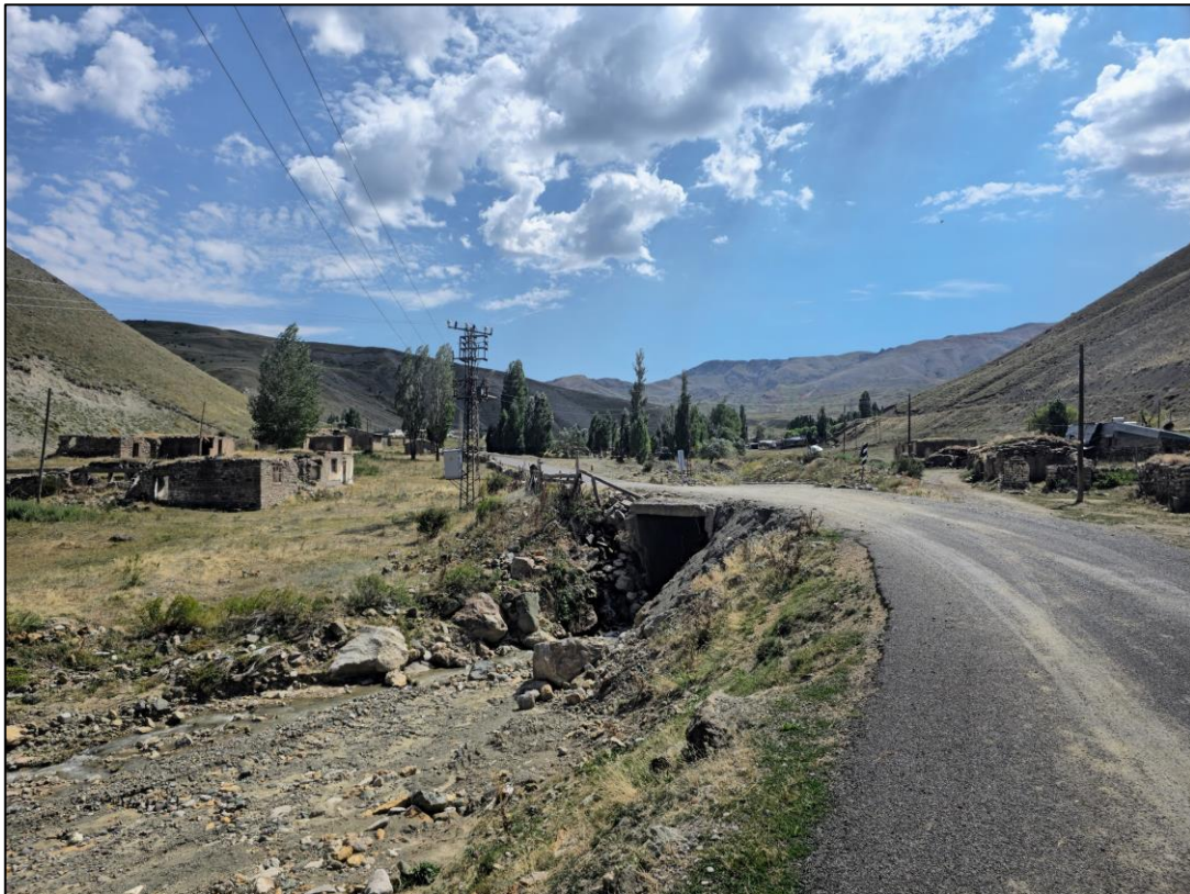
Figure 3: The Saçlık Village Center, where the flood occurred.
