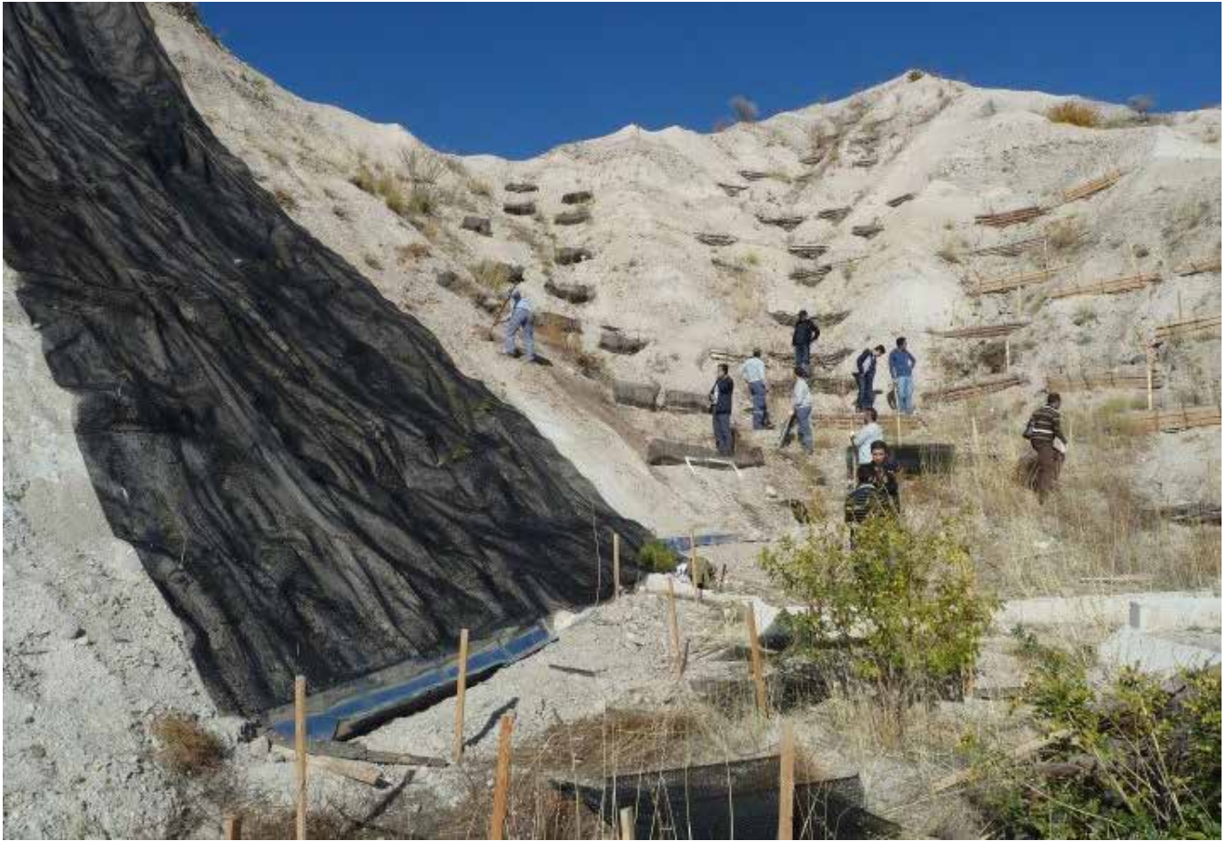
Figure 7. The application of geonet
