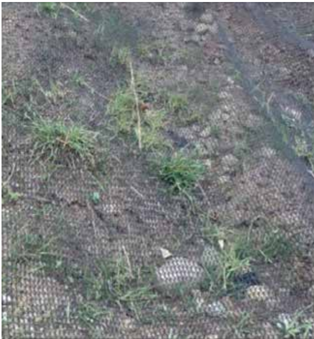
Figure 8. Start up of germination under the geonet
