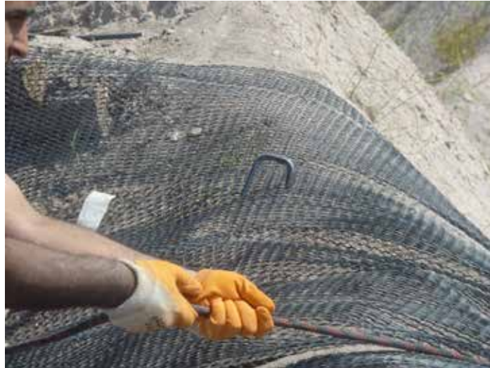
Figure 5. Laying of Tieback Anchors
