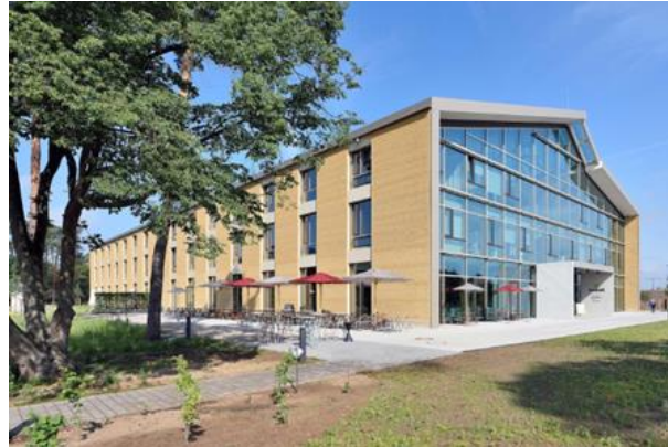
Figure 8. Image of the building (Url-4).
