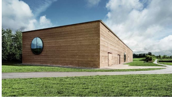
Figure 9. Image of the building (Url-6).
