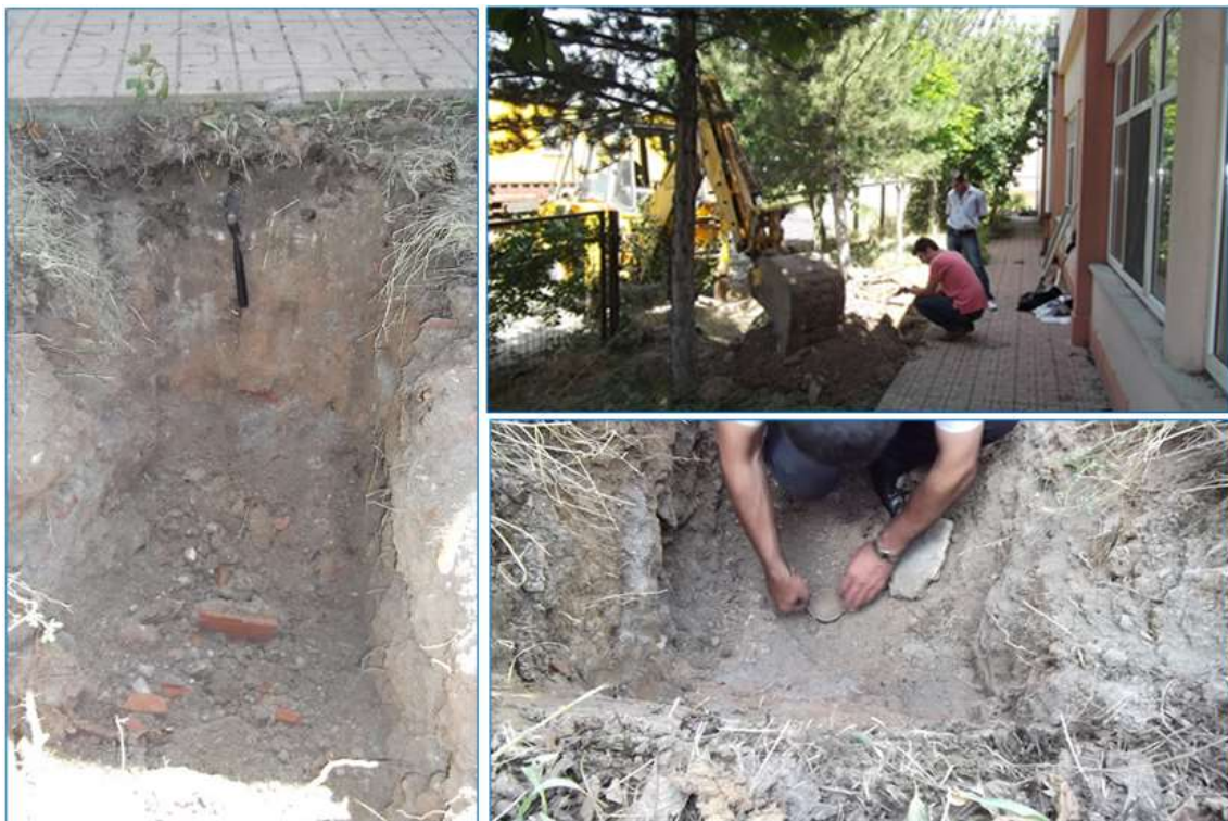
Fig. 10. View of the fill material from Trial pit-1 and undisturbed sampling
