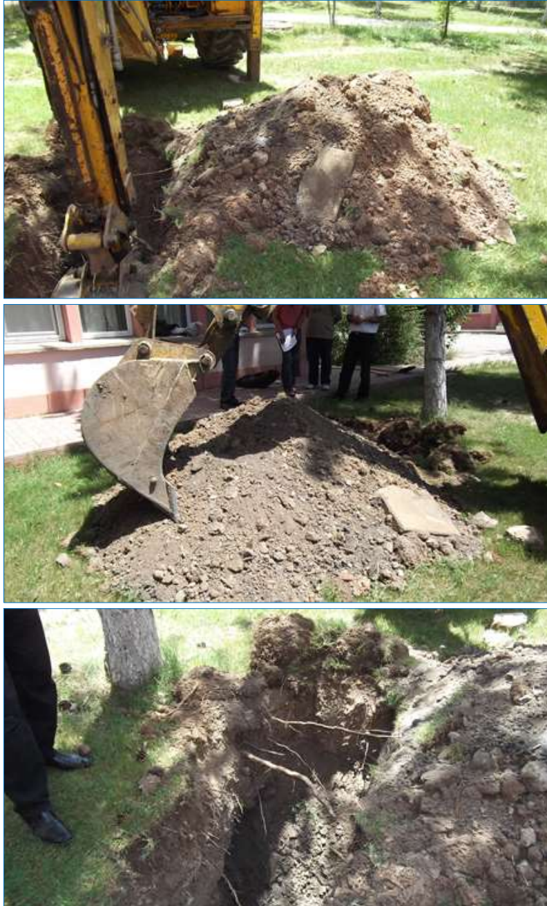
Fig. 13. Condition of the fill material from Trial pit-3
