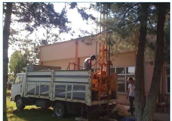
Fig. 9. A view of the drilling operation
