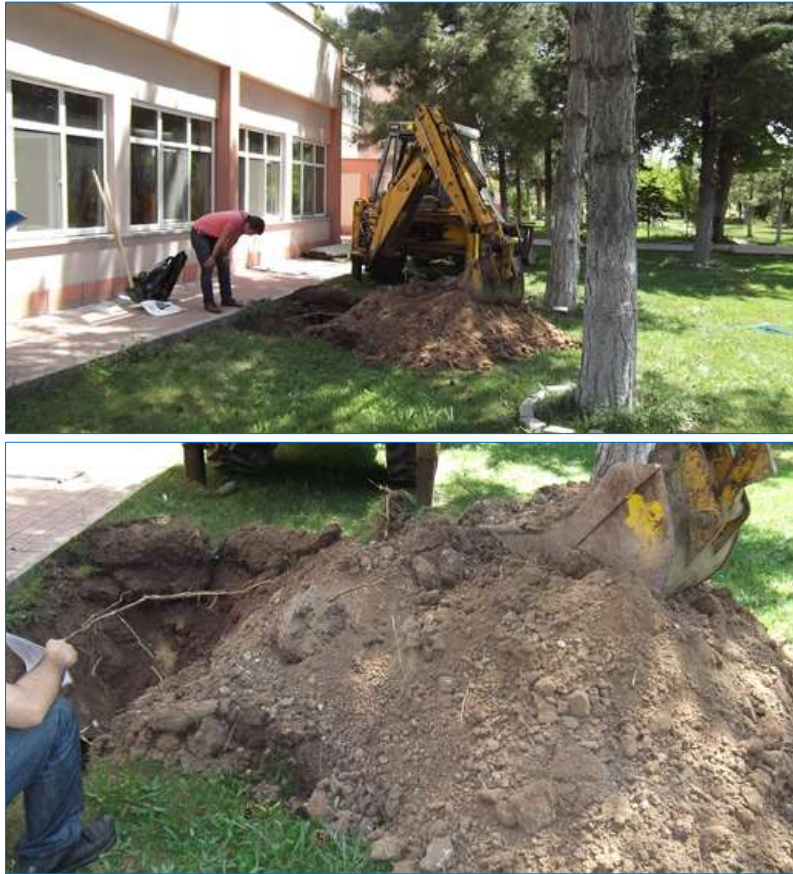
Fig. 11. Condition of the fill material from Trial pit-2
