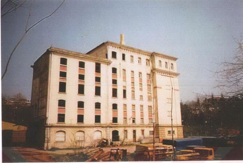
Figure 6. Nektar Beer Factory General View (Büyükdere Nektar Beer Factory Restoration Project)
