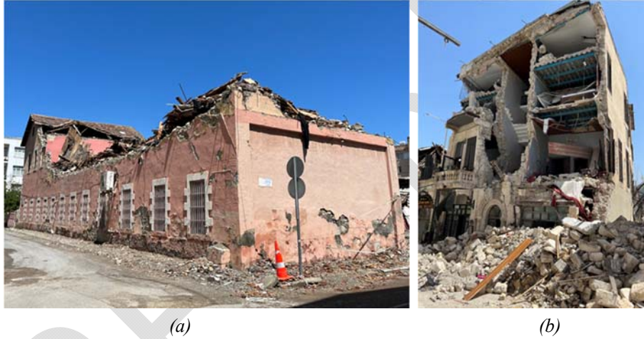
Figure 1 - Post-earthquake conditions of the analyzed URM buildings: (a) Mithatpaşa Primary School, Iskenderun, and (b) Liwan Boutique Hotel, Antakya.
