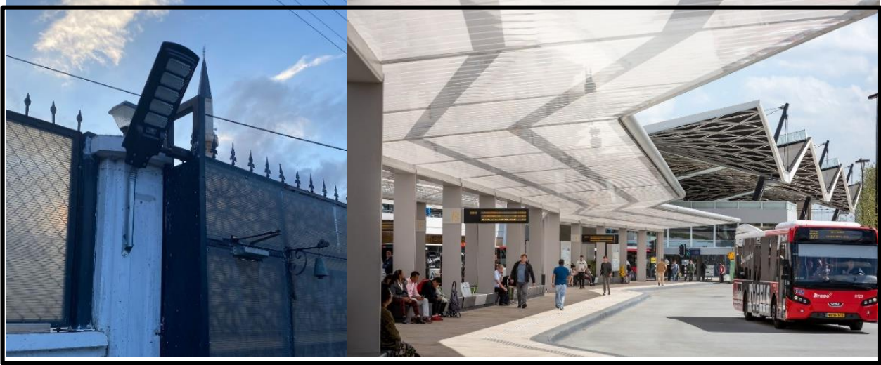
Figure 2. a- Solar powered lighting (Original, 2023), b- Solar-powered bus shelter (Wee, 2019)
