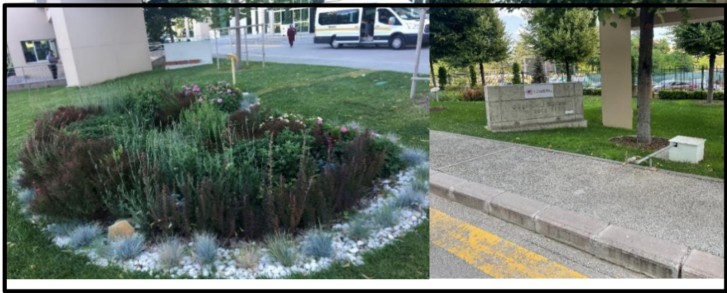
Figure 3. a- Rain garden application (Original, 2019), b- Permeable flooring application (Original, 2021)
