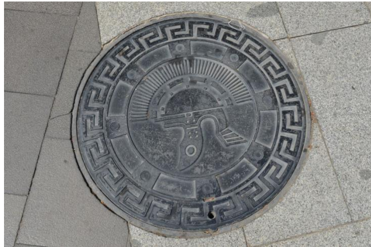
Figure 7. The drain covers used in the complex.
