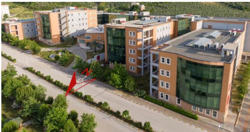
Figure 2. Aerial view of the building
