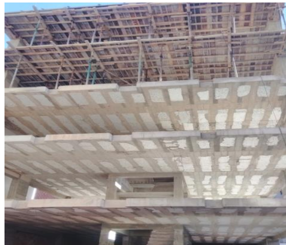
Figure 1. A building with hollow block slab
