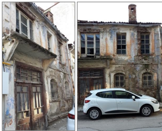
Figure 6. Front facade of the building (Created by the author)
