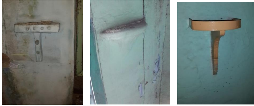
Figure 8. Original plaster and inappropriate accretion metal ırappas (niches for lamps) from rooms M-02, M-04 and Z-01 (Created by the author)
