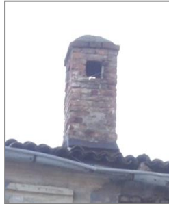
Figure 9. The original brick chimney of the building (Created by the author)
