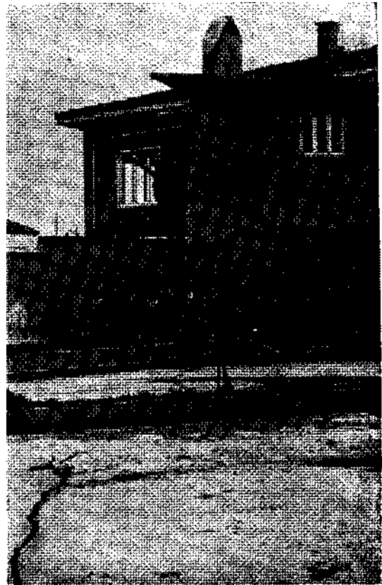
Photo 8 - Fracture number 2 crossing one of the main streets in Alaqehir Village. Northern block (left-hand side) is depressed.
